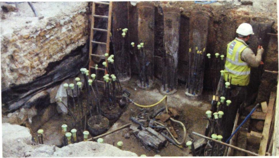
Figure 3.06 Cutting down pile heads to formation level
