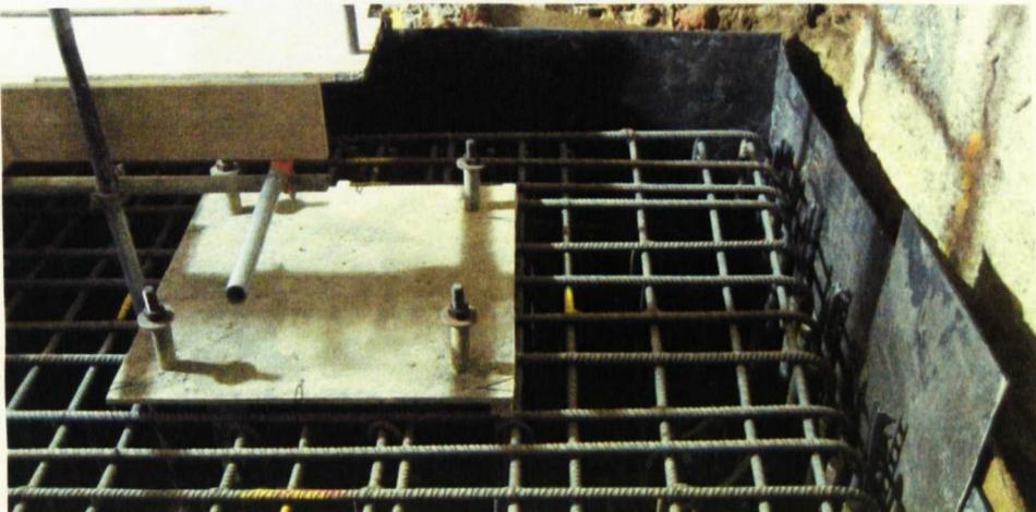
Figure 3.08 Installation of structural column connection plate
