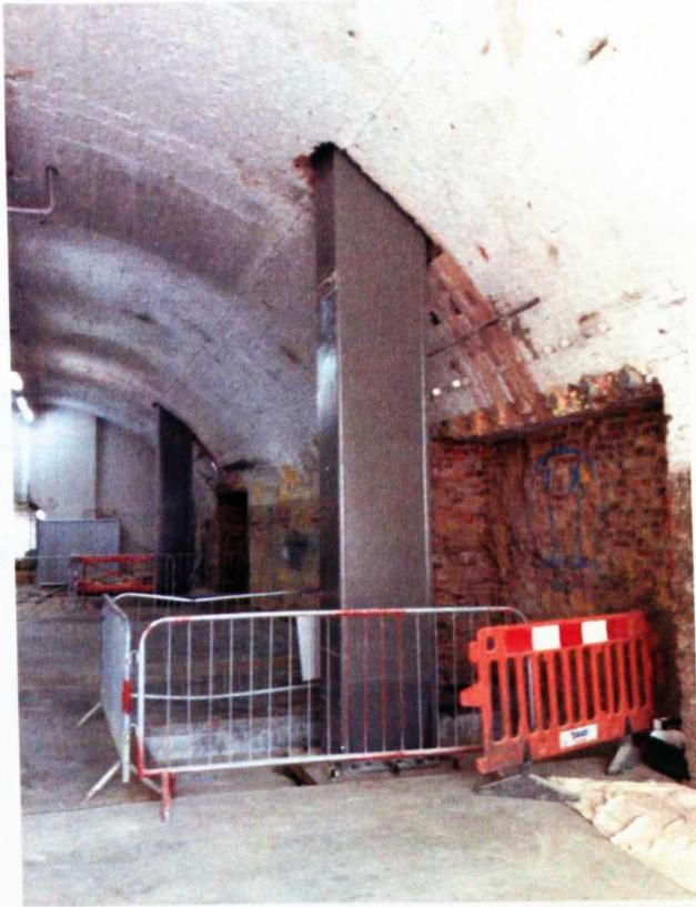
Figure 3.11 Structural column installed
