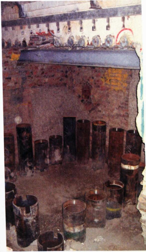
Figure 3.04 Piles installed through casing
