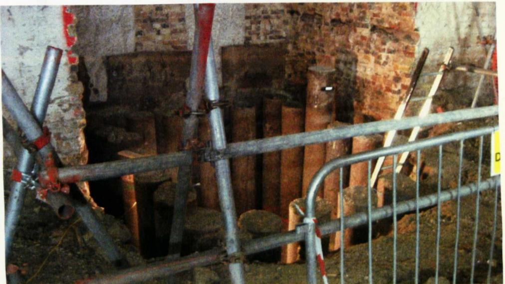
Figure 3.05 Excavation to pile cap formation level
