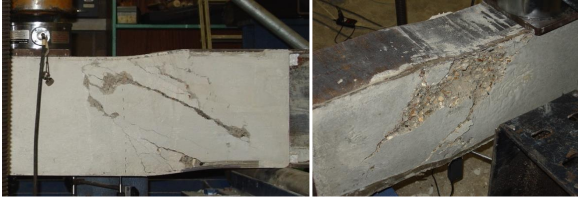
Fig. 11: USFB No.3 with concrete bursting
