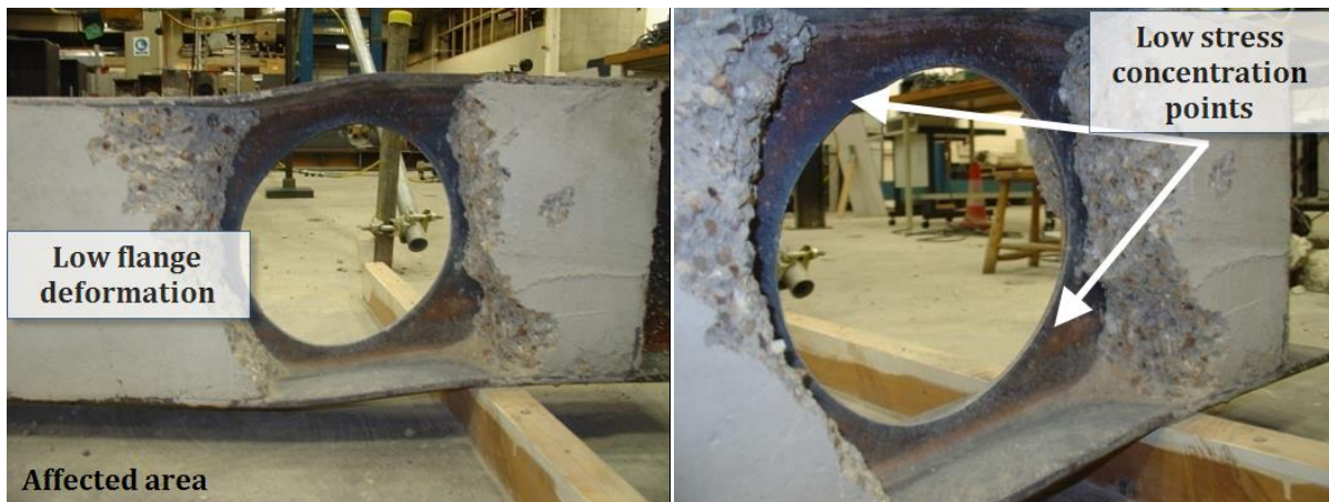
Fig. 13: Failure mode for partially encased USFB No.1 at opening after removal of the damaged concrete
