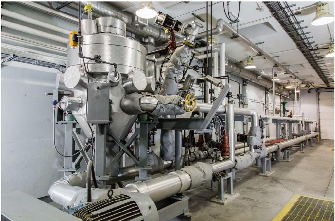
**Figure 3.2 Closed loop pumping system (SASKATCHEWAN RESEARCH COUNCIL, 2014)**
