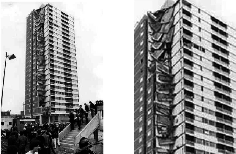
Fig. 2.1 Disproportionate collapse of Ronan Point (Pearson and Delatte, 2005)
