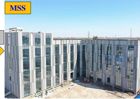
(c) Corner-supported modules with shear-keyed grouped tubes in the MSS project in China (Designed by the research team) [68]
