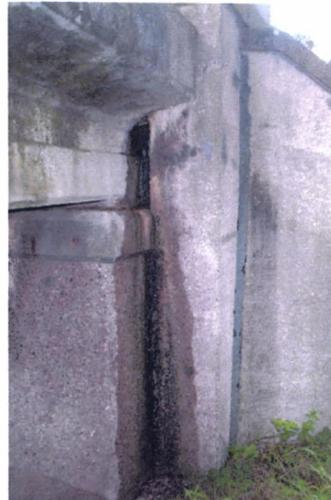
**Figure 7.2** Abutment area showing exposed reinforcement
