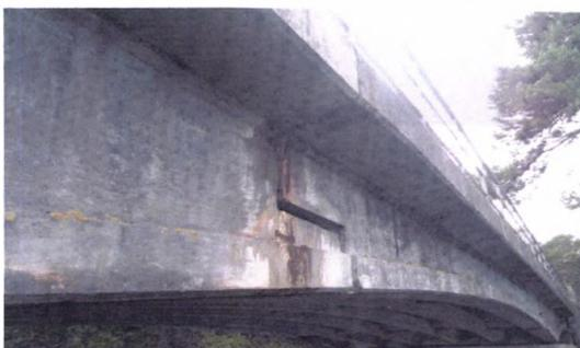
**Figure 7.3** Half joint showing rust staining at bearing
