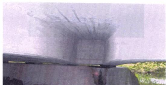
**Figure 7.4** View of bearing plinth showing concrete spalling
