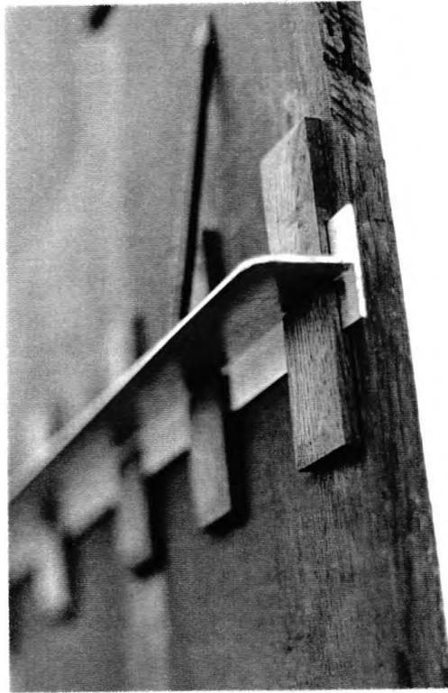
Figure 13. A T-section aluminium sliding batten.
