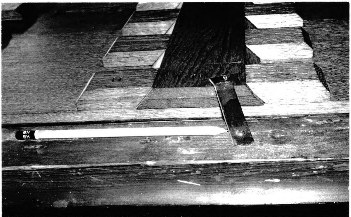
Figure 25. A laminated panel. The panel has been thinned to about 1mm (darker layer above pencil), laminated to thicker oak planks, then reinforced further with relatively rigid sliding oak battens.
