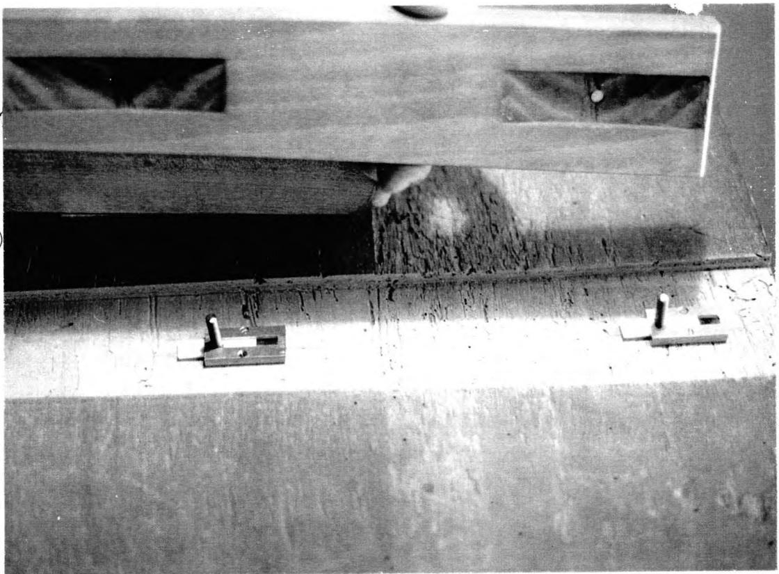
Figure 16. A rigid sliding batten with retainers sprung to allow for warp movement: a) batten with flat spring-steel rectangles in place and bolted into groove in panel back, b) batten removed, showing outer face with depressions for springs, brass retainers screwed to panel, and sliding mechanisms consisting of bolts trapped in low-friction plastic strips.
