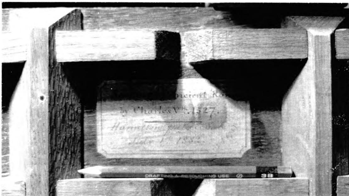
Figure 10. Detail of what is probably a 19th c. "Italian cradle". A paper label from an Italian exhibition is dated 1882. It's position between the sliding battens indicates it was applied after the battens.
