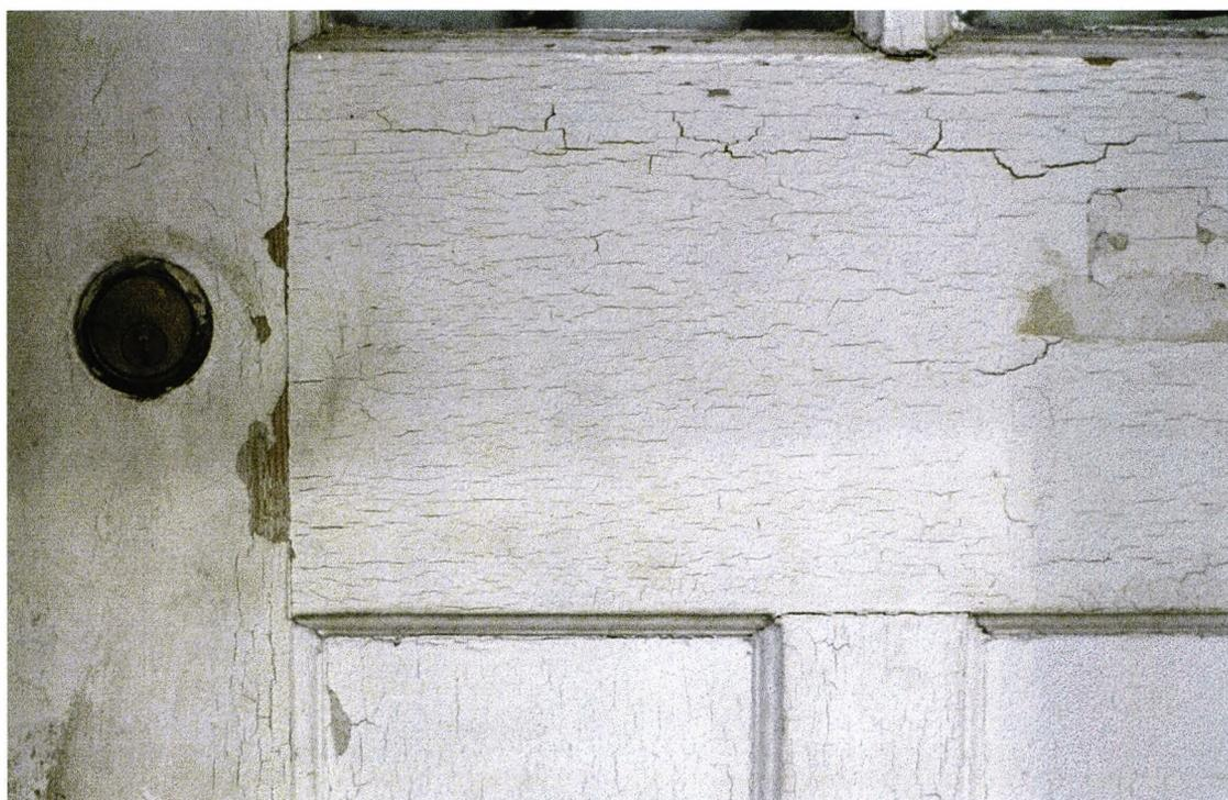
Figure 2.3. Cracking predominately along the grain and direction of brush strokes on this wooden house front door. If the coating had been sprayed onto a substrate with no grain, the cracking would tend to be hexagonal. Some accidental damage can be seen around the lock rose. This could account for the localised flaking.
