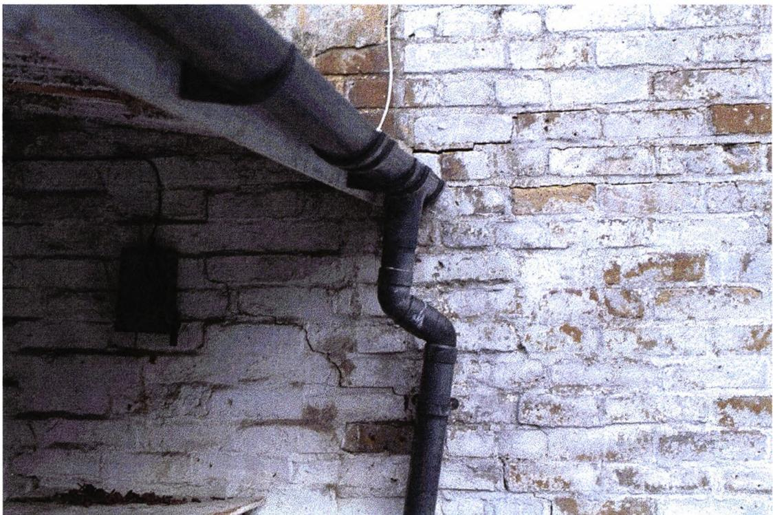
Figure 2.2. The sheltered part of the wall to the left has become soiled, but the paint is intact. On the right, the wall is not roofed. Rain has cleaned the black dust from the pointing, but the coating has failed .
