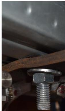
Bolted studs' failure.
