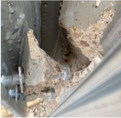
Concrete cone failure.
