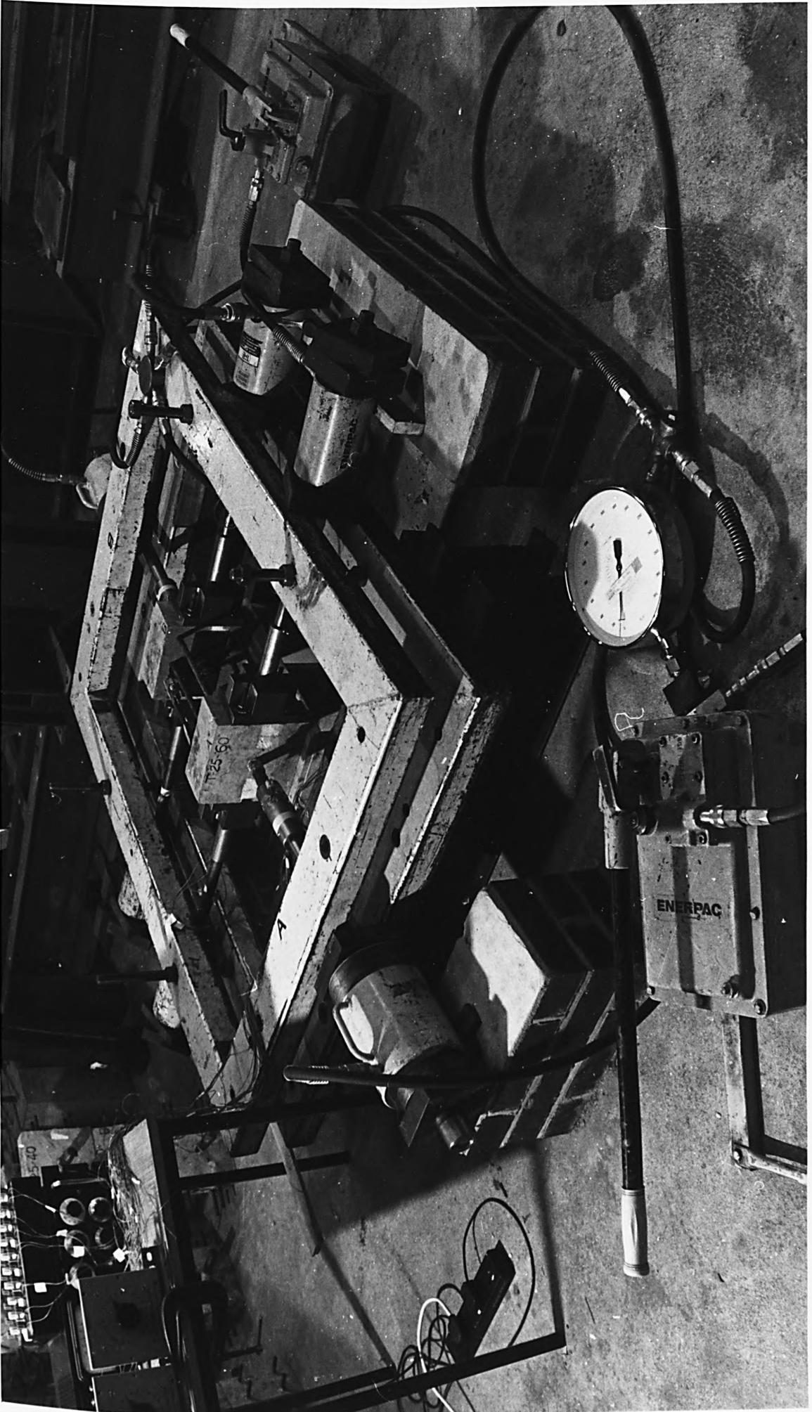
FIG. 3.6 PHOTOGRAPH SHOWING BOND TEST UNDER LATERAL TENSION RELEASE
